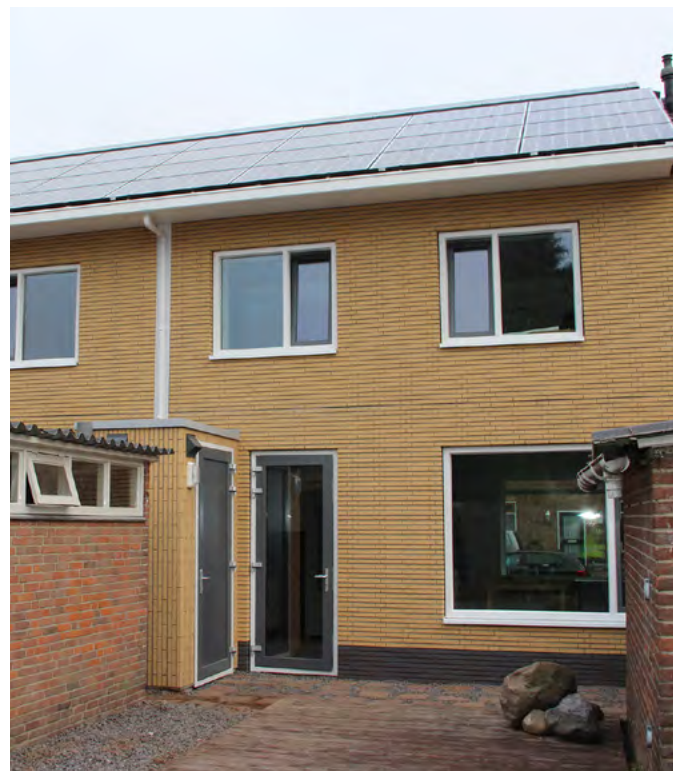
Ergieneutrale woning project Stroomversnelling te Soesterberg. www.stroomversnelling.net
